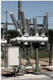
PASS hybrid switchgear
